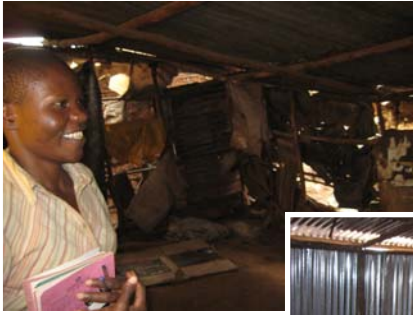
Inside the 10 x 14 feet KOPLWA centre in Kibera – Before (above, with mud floor and walls of cardboard and cloth) and after the improvement of the infrastructure (right, with concrete floor and more proper Ironsheet walls).
