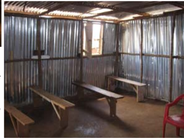
Inside the 10 x 14 feet KOPLWA centre in Kibera – Before (above, with mud floor and walls of cardboard and cloth) and after the improvement of the infrastructure (right, with concrete floor and more proper Ironsheet walls).
